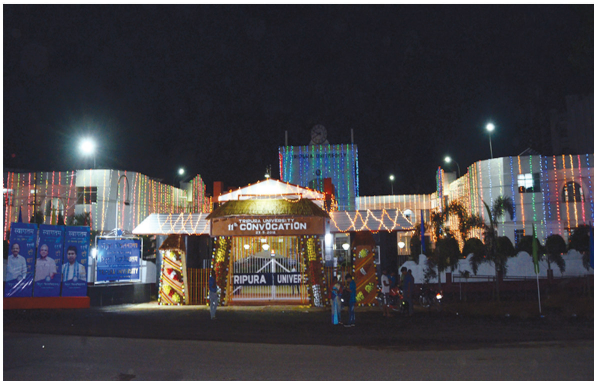
View of Tripura University Administrative Building
